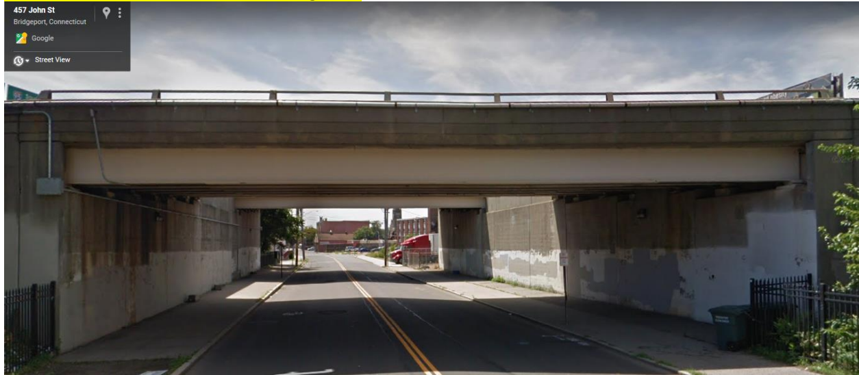
#8-C: Rt 8/25 and John Street, looking west
