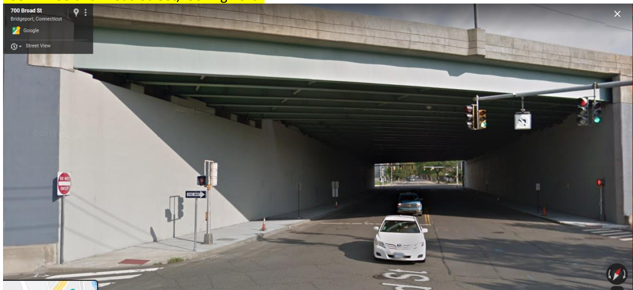
#95-E: I-95 and Broad Street, looking north
